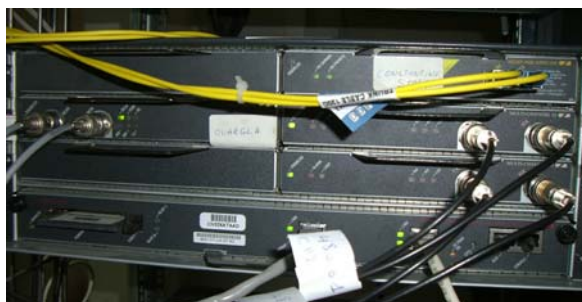
Photo from EUMEDCONNECT Algeria: Interconnection through circuit with Spain with the International NREN community and distribution to the local Points of presence in Algeria
