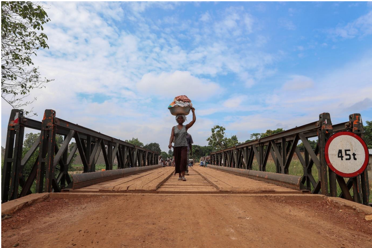
Figure 8. Pont Bailey installé
