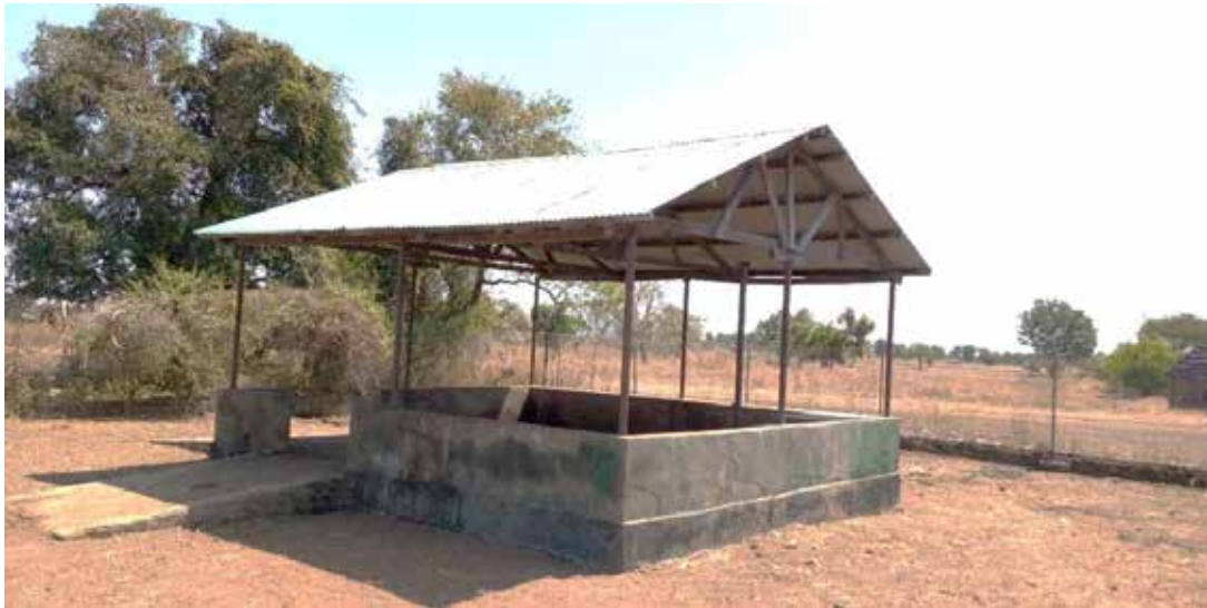
Figure 2: Slaughter slab constructed at Malek Alel in 2008
