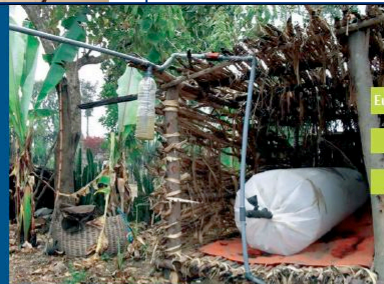
Plastic biogas plant
