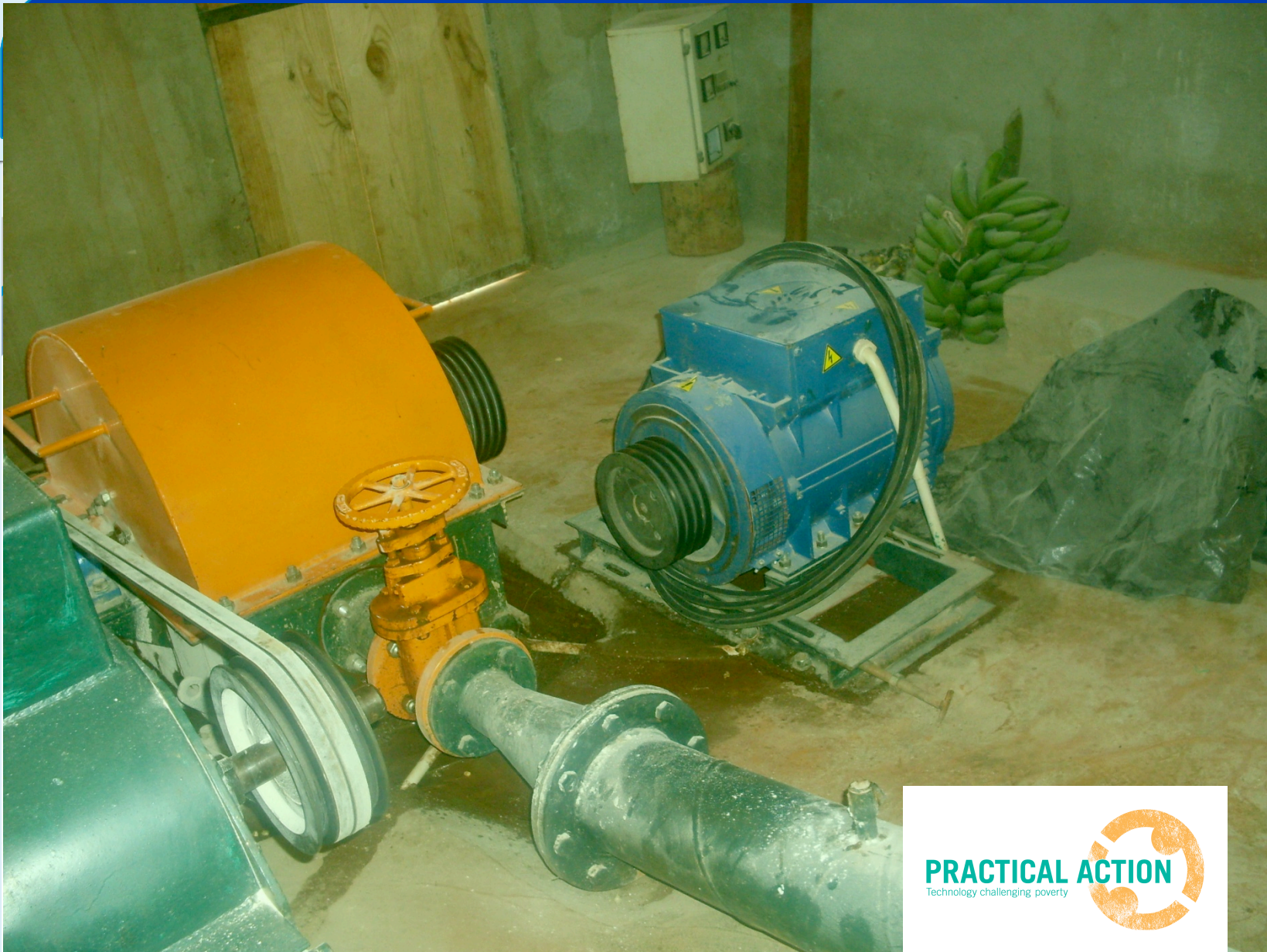
Coupling Arrangement of Generator, Turbine and grinding mill at Ndiriri, Manica.
