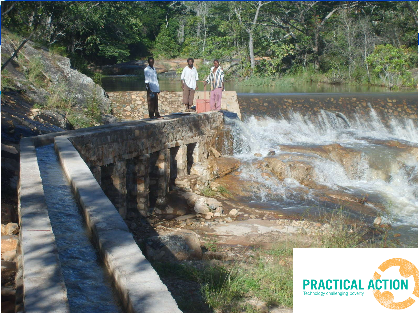
Completed weir and lined canal at Chipendeke, Mutare.
