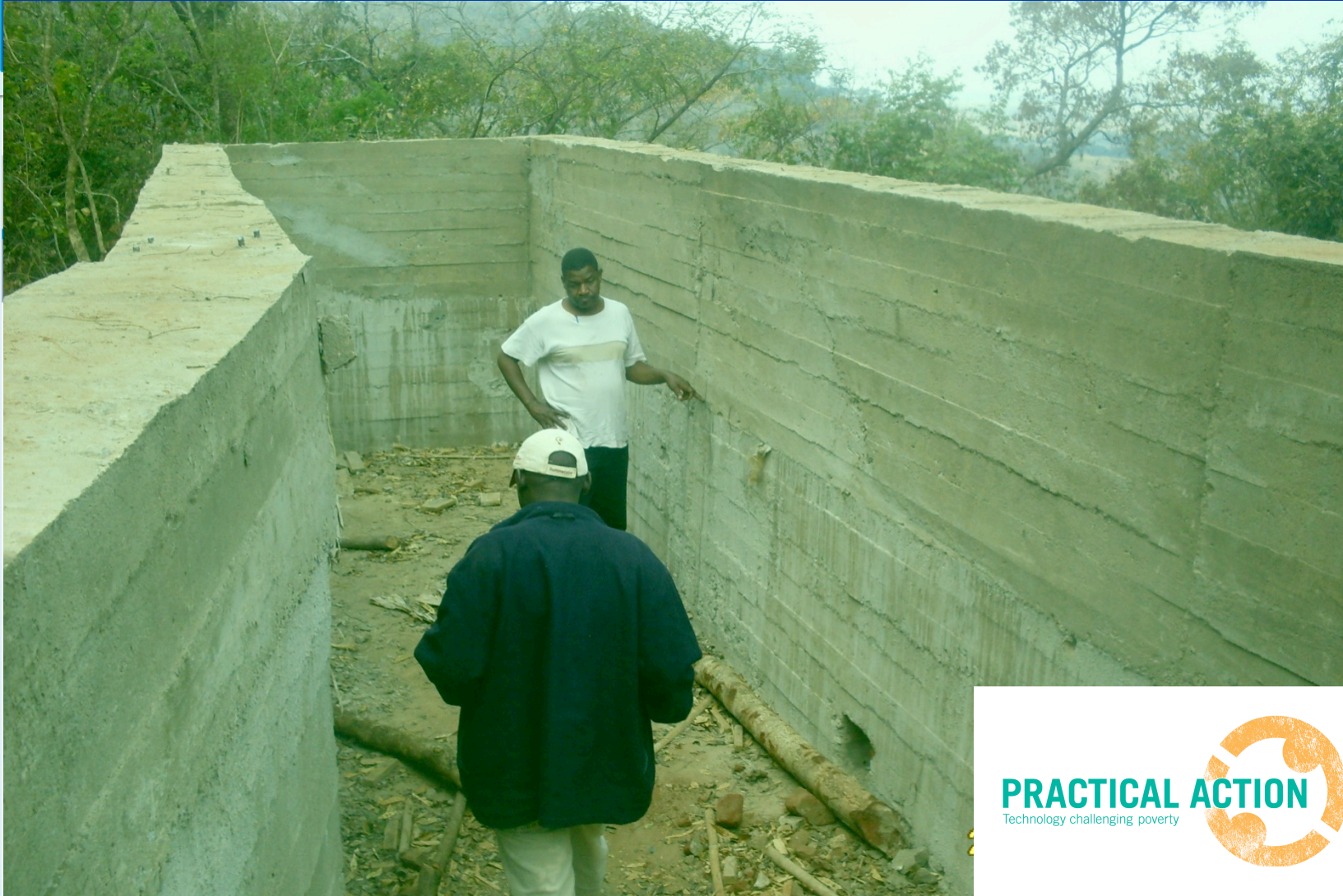
Forebay and two desilting Tanks at Chitunga, Manica.
