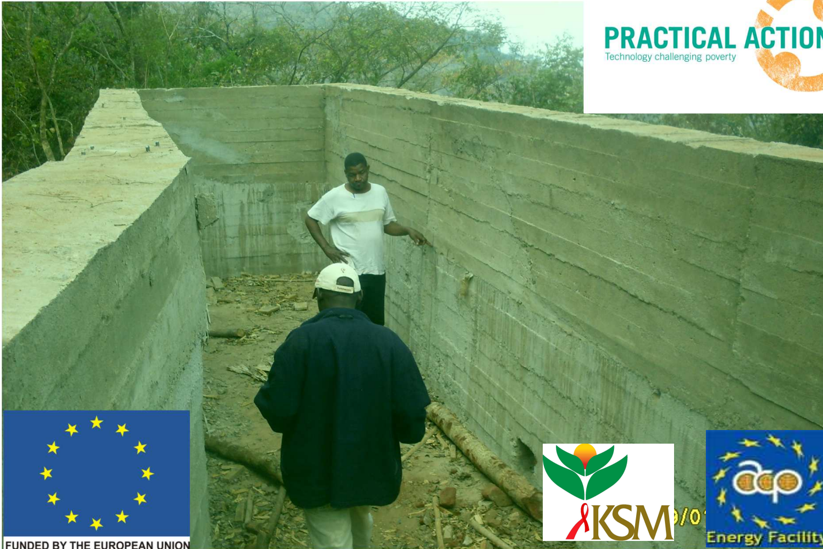
Forebay and second desilting Tank at Chitunga, Manica.
