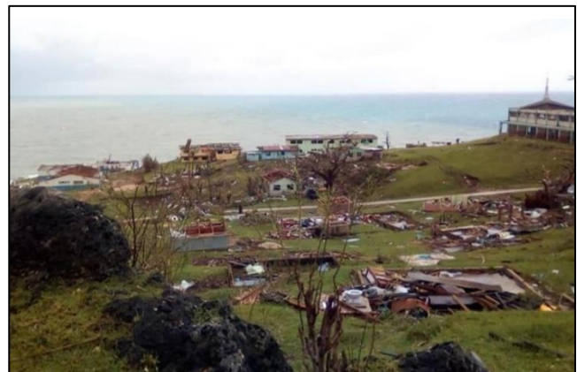
Destruction in Vanuatu following tropical cyclone Harold.
