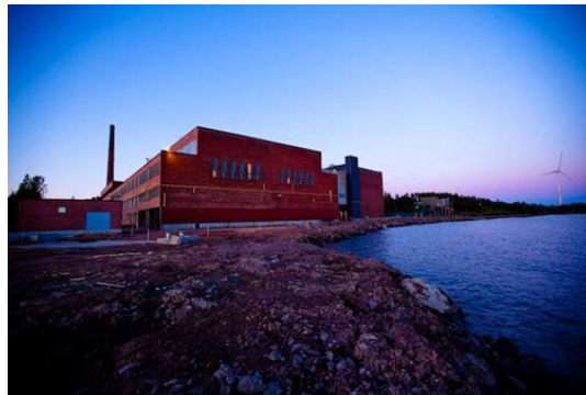
Figure 10.10. Google data center opened in 2011 in Hamina, Finland (left) with closed-loop water cooling (right). Source: ©2018 Google LLC, used with permission. Google and the Google logo are registered trademarks of Google LLC
