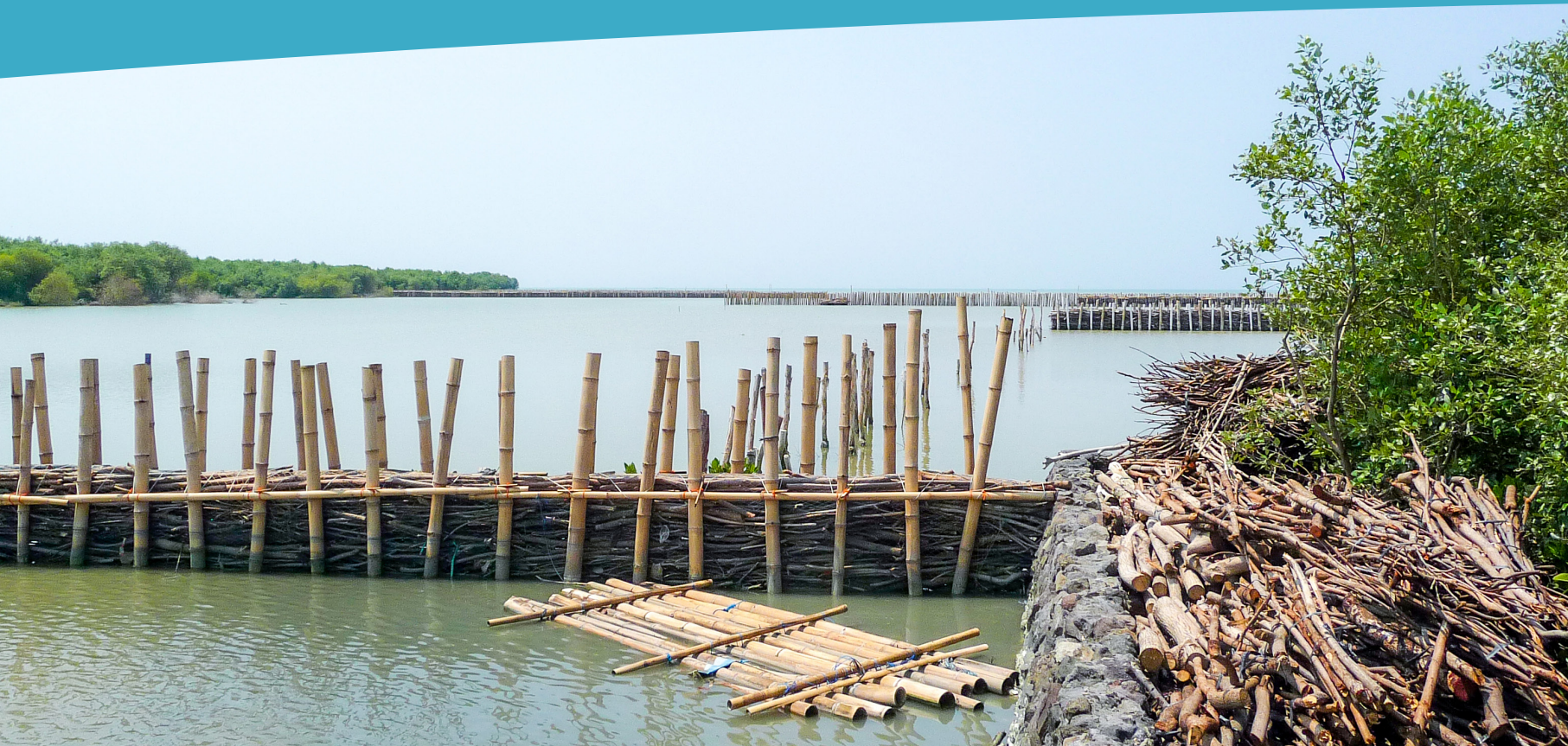
Figure 1. Permeable structures in Timbulsloko (Demak, Indonesia) © Tom Wilms, Witteveen+Bos
