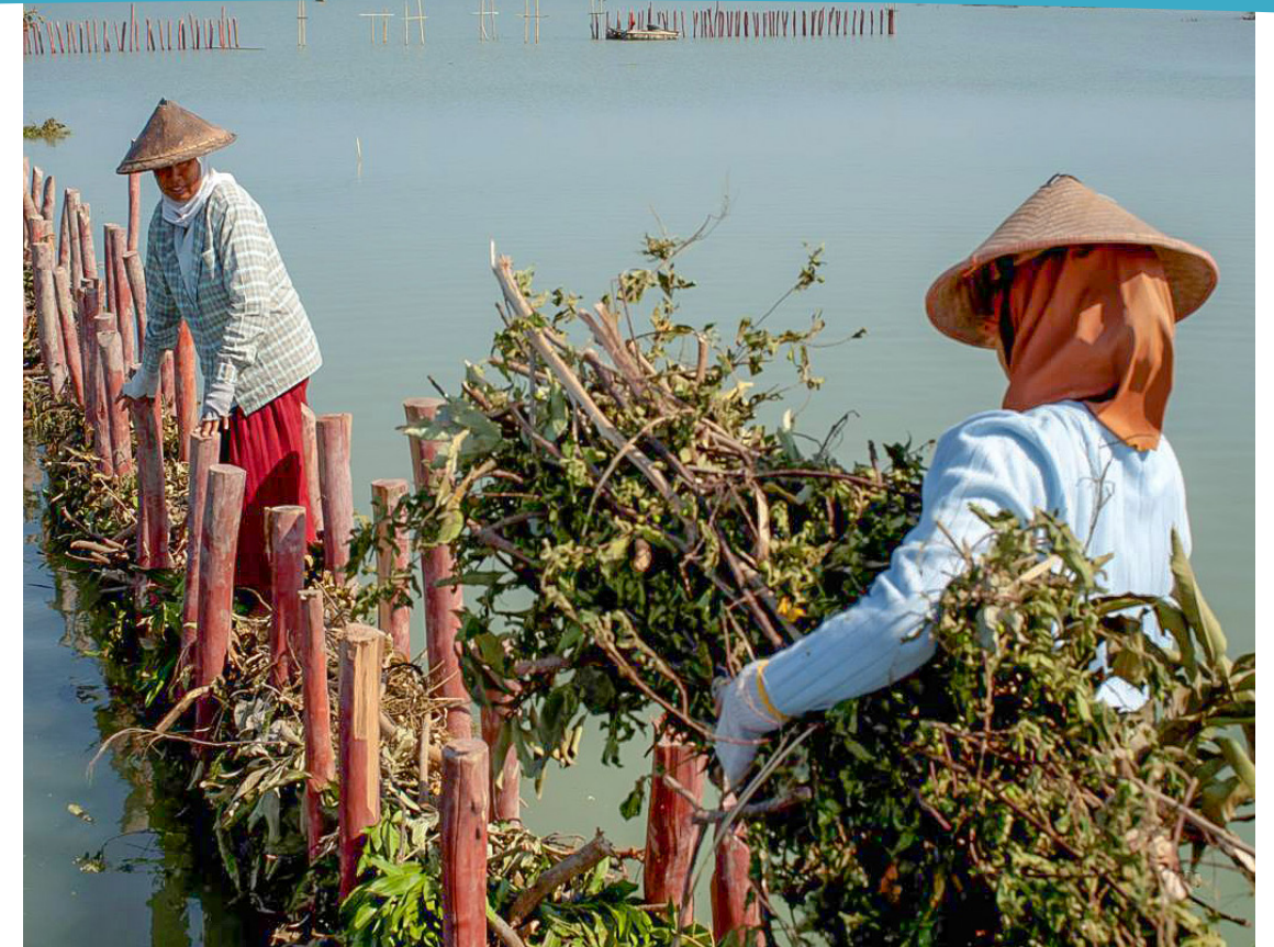
Figure 2. Construction of permeable structures by local women in Timbulsloko (Demak, Indonesia) © Nanang Sujana
