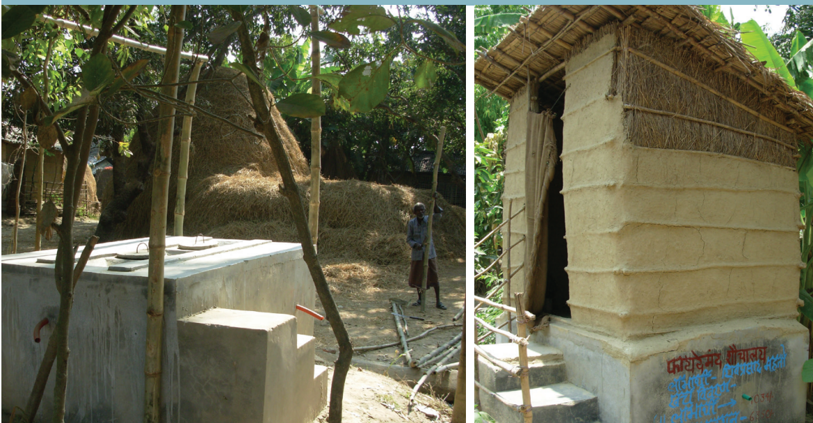
This project in Bihar, India, tackled the financing issue by providing the concrete substructure for flood-resistant toilets, while households were responsible for building the superstructure. Photo: Kim Andersson
