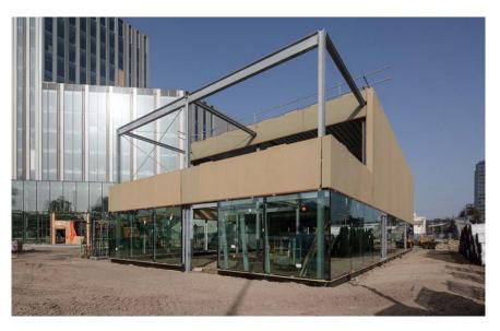
façade consists of the glass of the old Knoopkazerne; the glass size determined the dimensions of the pavilion
