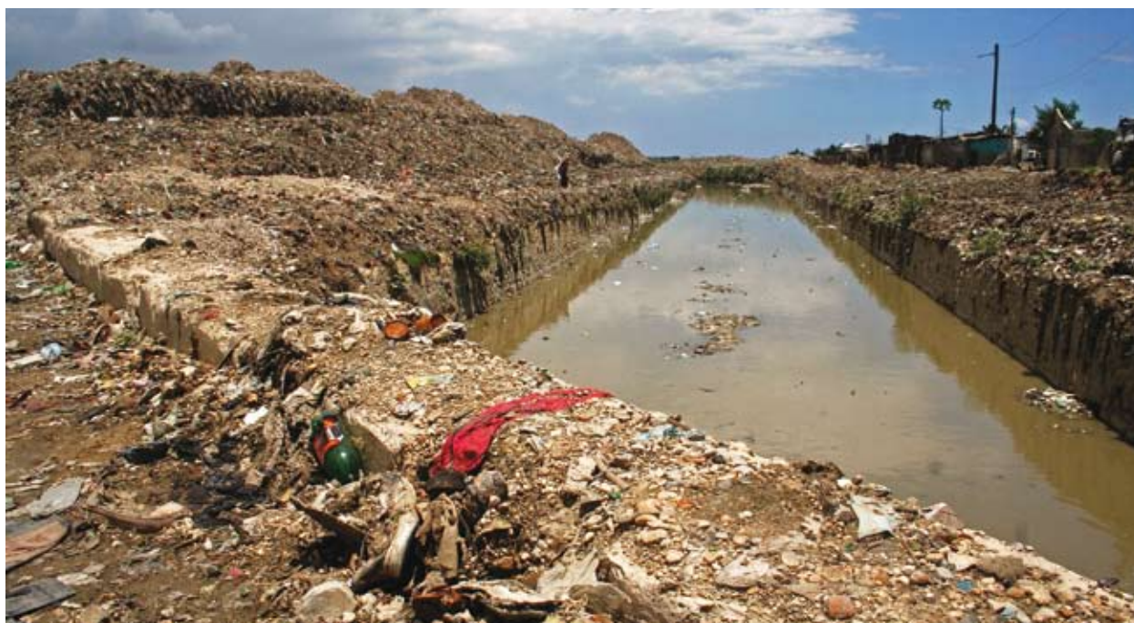
The severely polluted and blocked drainage canals in Port-au-Prince are a chronic source of infections and prone to flooding
