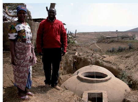
Biogas digester built thanks to the Best Buy (Bringing energy services to Tanzanian rural areas) project
