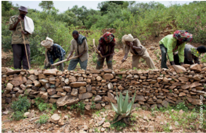
Stone terraces for soil and water conservation in Ethiopia
