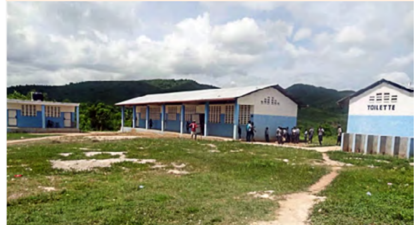
Source: Janice Rodgers, GeoHazards International – Rapid diagnostic of school infrastructure in Haiti (unpublished)
