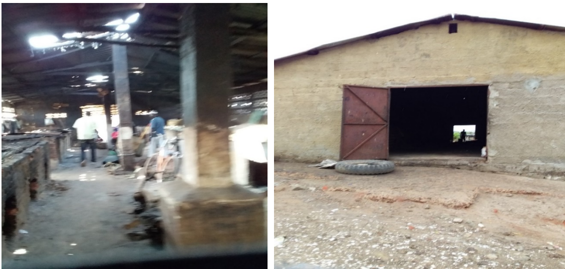
FIGURE 28. OVENS AND SMOKEHOUSE
