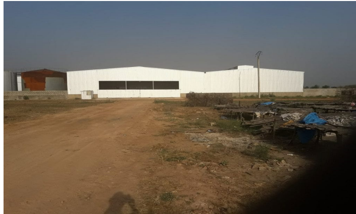
FIGURE 31. LOCATION OF A FACTORY IN GUNJUR ON AN ARTISANAL PROCESSING SITE
