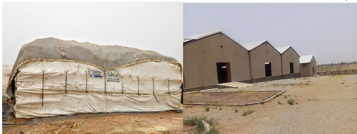
FIGURE 17: DIFFERENT GRAIN STORAGE FACILITIES IN THE KADUNA STATE (2020)
