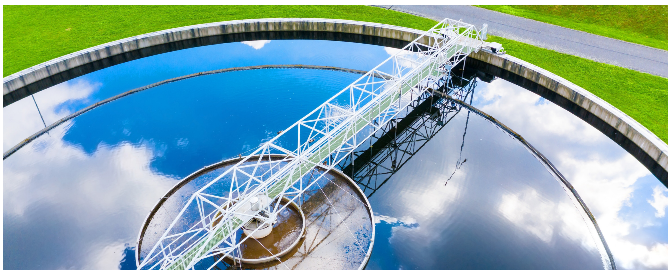
Wastewater treatment tank. Source: Shutterstock.
