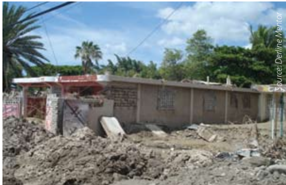
Figure 81: Gonaives in the aftermath of the 2008 hurricanes
