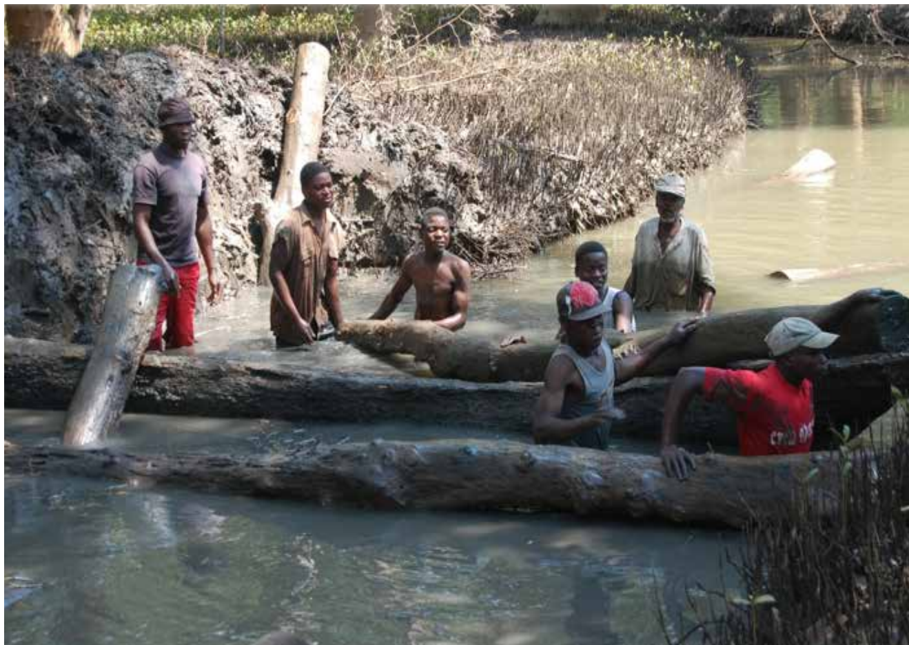
COMMUNITY MEMBERS PARTICIPATING IN THE CONSTRUCTION OF SMALL DAM TO REGULATE WATER FLOW TO MANGROVE REFORESTATION AREA
