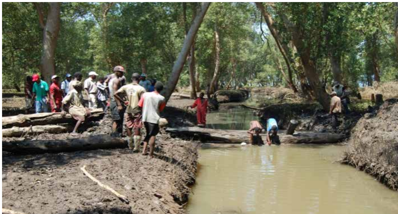
COMMUNITY MEMBERS PARTICIPATING IN THE CONSTRUCTION OF SMALL DAM TO REGULATE WATER FLOW TO MANGROVE REFORESTATION AREA
