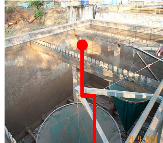
Old clarifiers before rehabilitation
