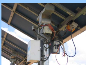
Detail of connection between solar tracking array and controller
