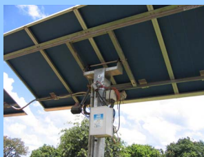
Panels on solar tracking array
