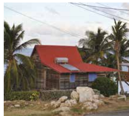
Image: Kate Shifman | Barbados, Solar Water Heater
