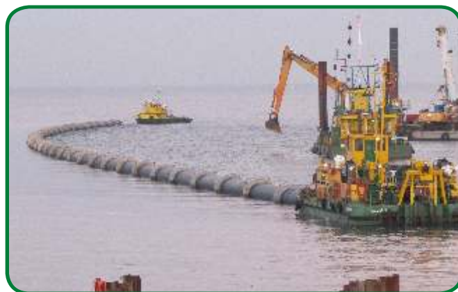
„Underground pipe installation” Photo: Gmina of the Town of Sopot
