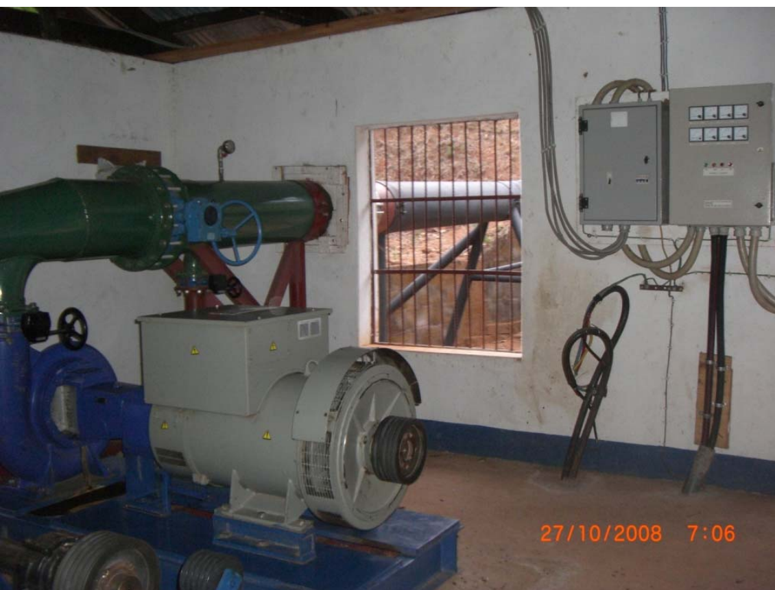
Turbine, generator & Control panel
