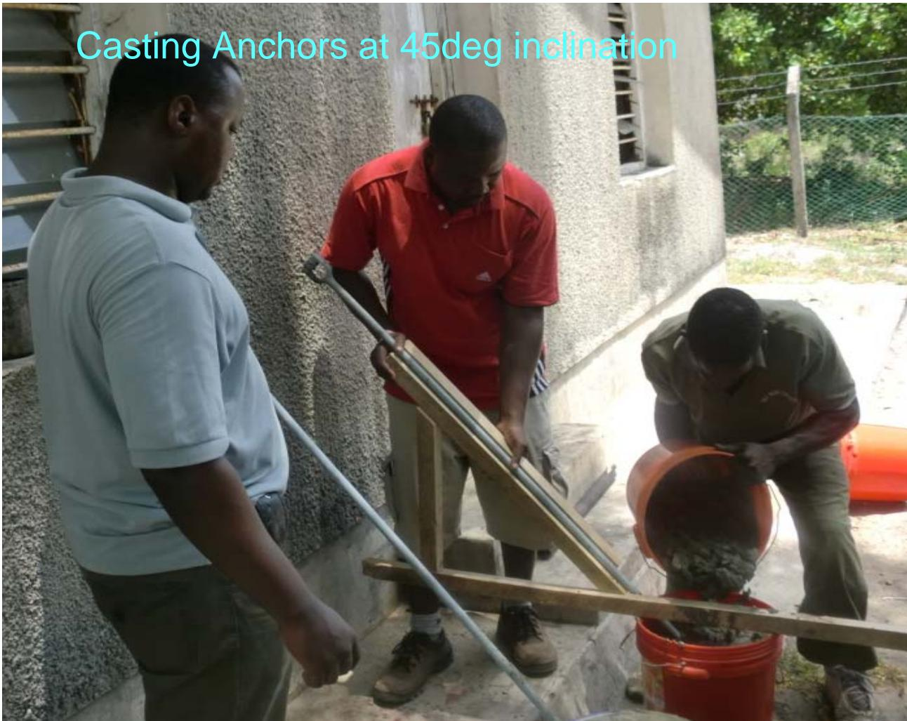
Casting Anchors at 45deg inclination
