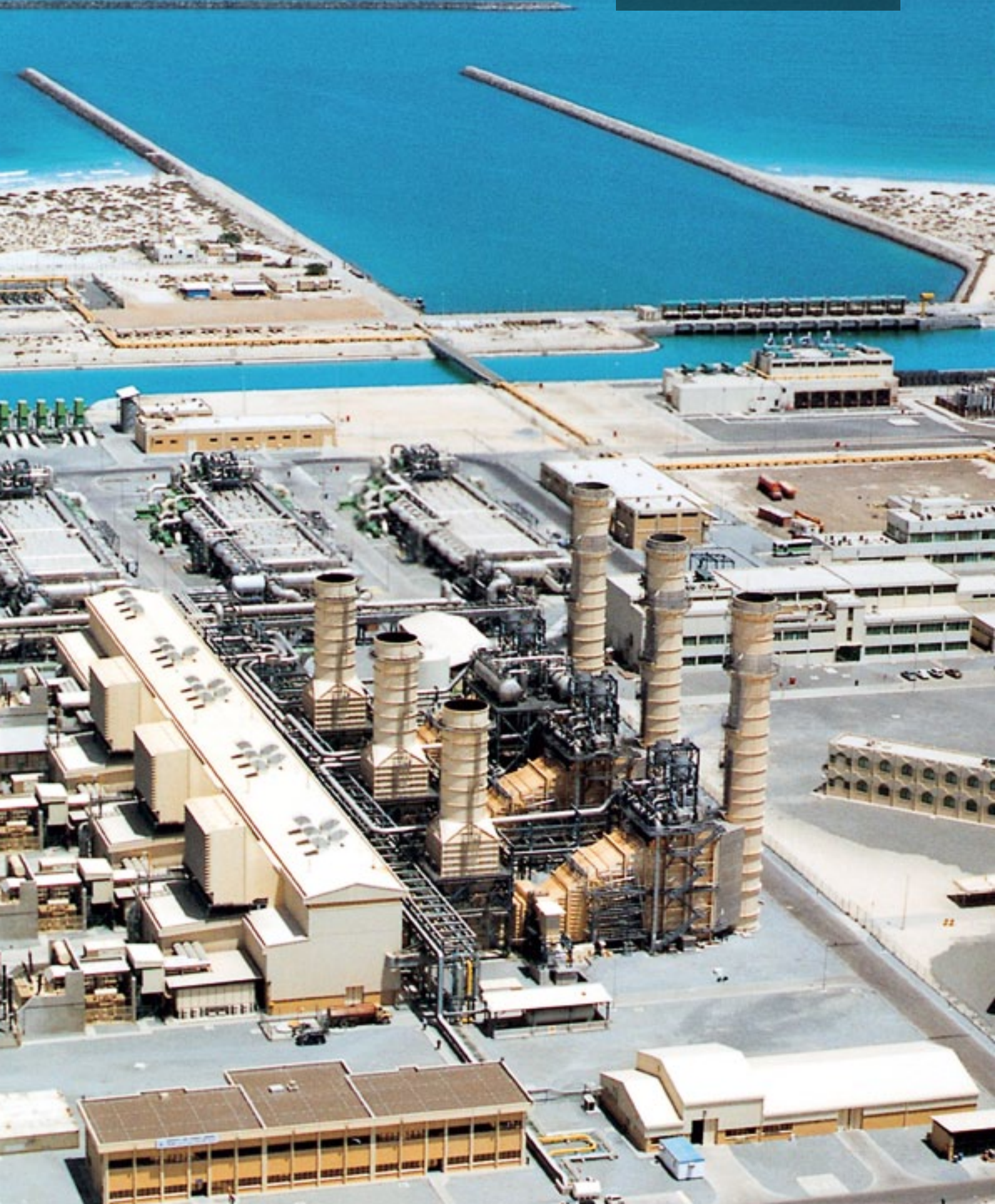
Al Taweelah A2 gas and steam power station and a connected desalination plant in the United Arab Emirates
