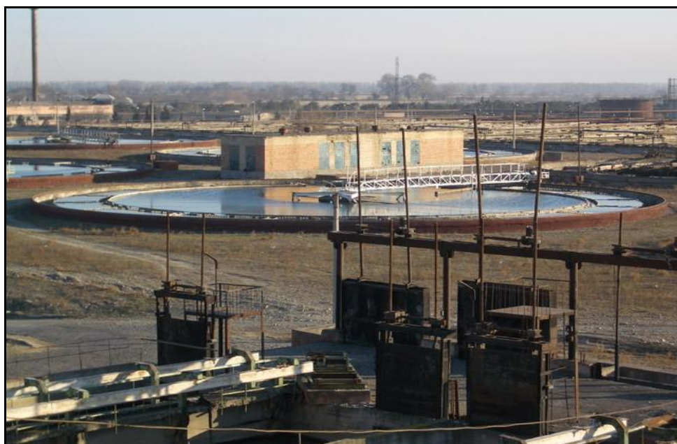
Figure 10. Picture 0-1 Sand traps and primary sedimentation tanks on Gardabani WWTP in operation
