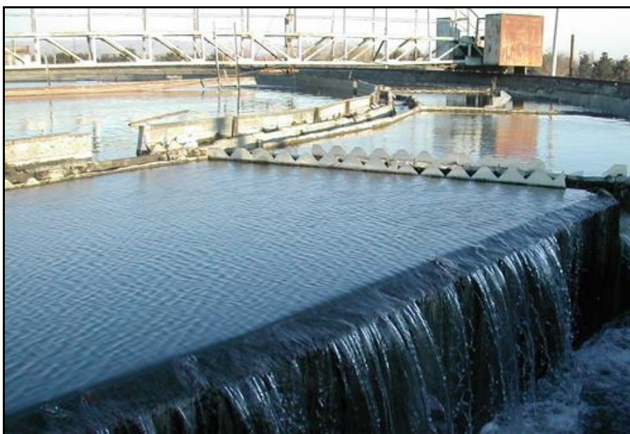
Picture 0-3 Primary radial sedimentation tank in operation. Overflow
