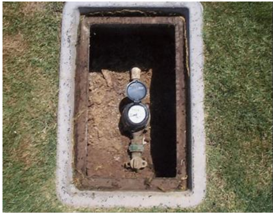
Install bulk water meters
