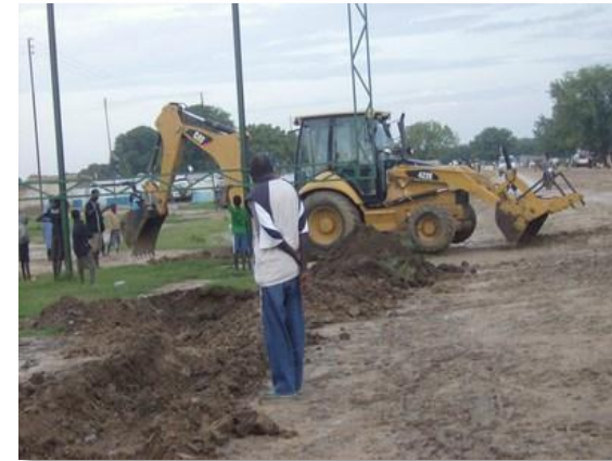
Repair visible leaks on the reticulation system
