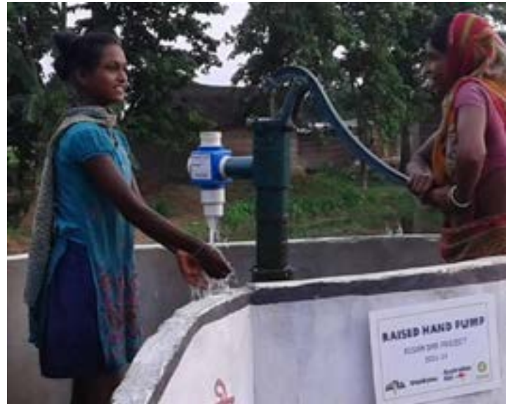
Figure 8. PurAll Handpump chlorinator (Source: EaSol Private Limited)
