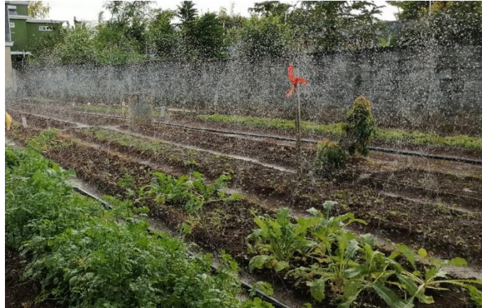
Novel irrigation system: KNSM spray irrigation system
