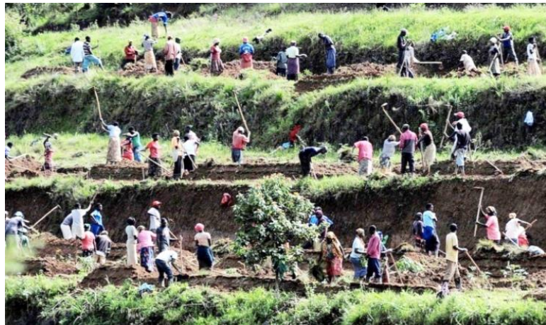
Maintenance of soil and water conservation structures (bench terraces) in fragile and marginal lands in Ethiopia. Photo credit: ASARECA
