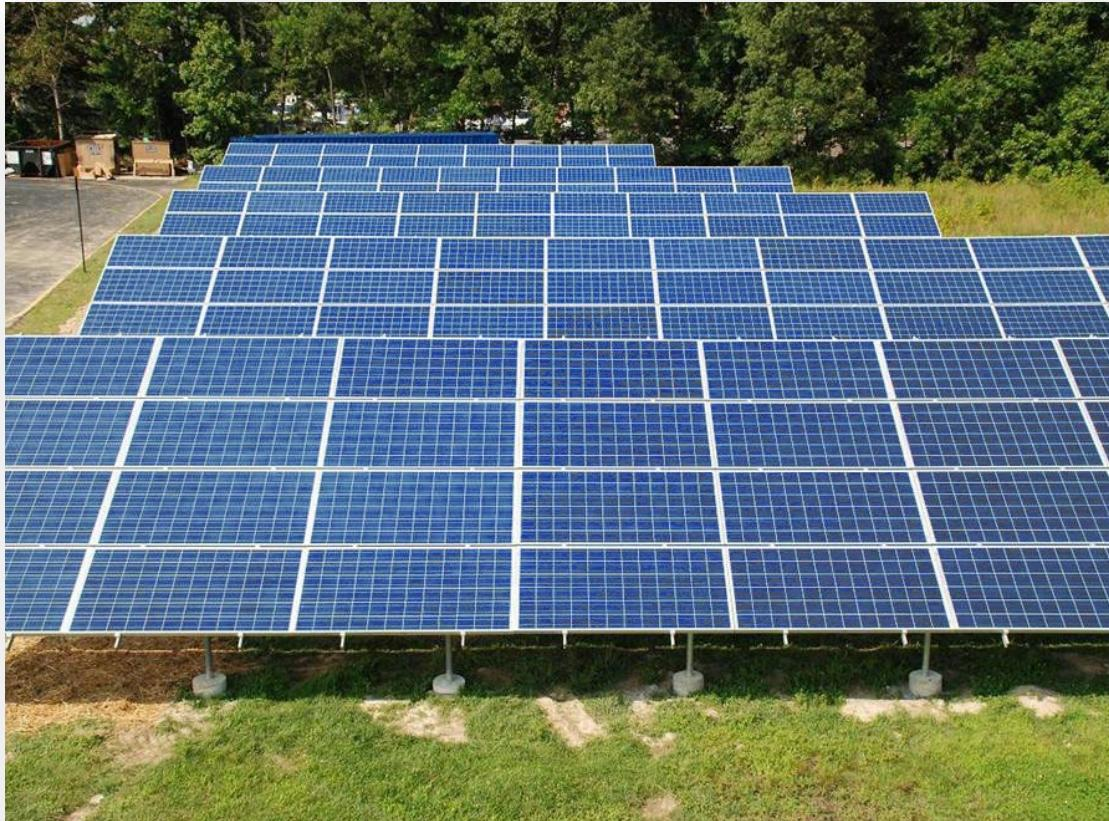
1 MW grid-connected, ground mounted solar PV project
