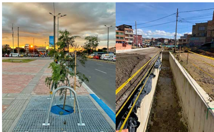
Figure 5.4: Floodable pits on Rincon Avenue, Suba, Bogota (left) and infiltration ditches with bioretention zones under construction on Rincon-Boyaca Avenue (right).
