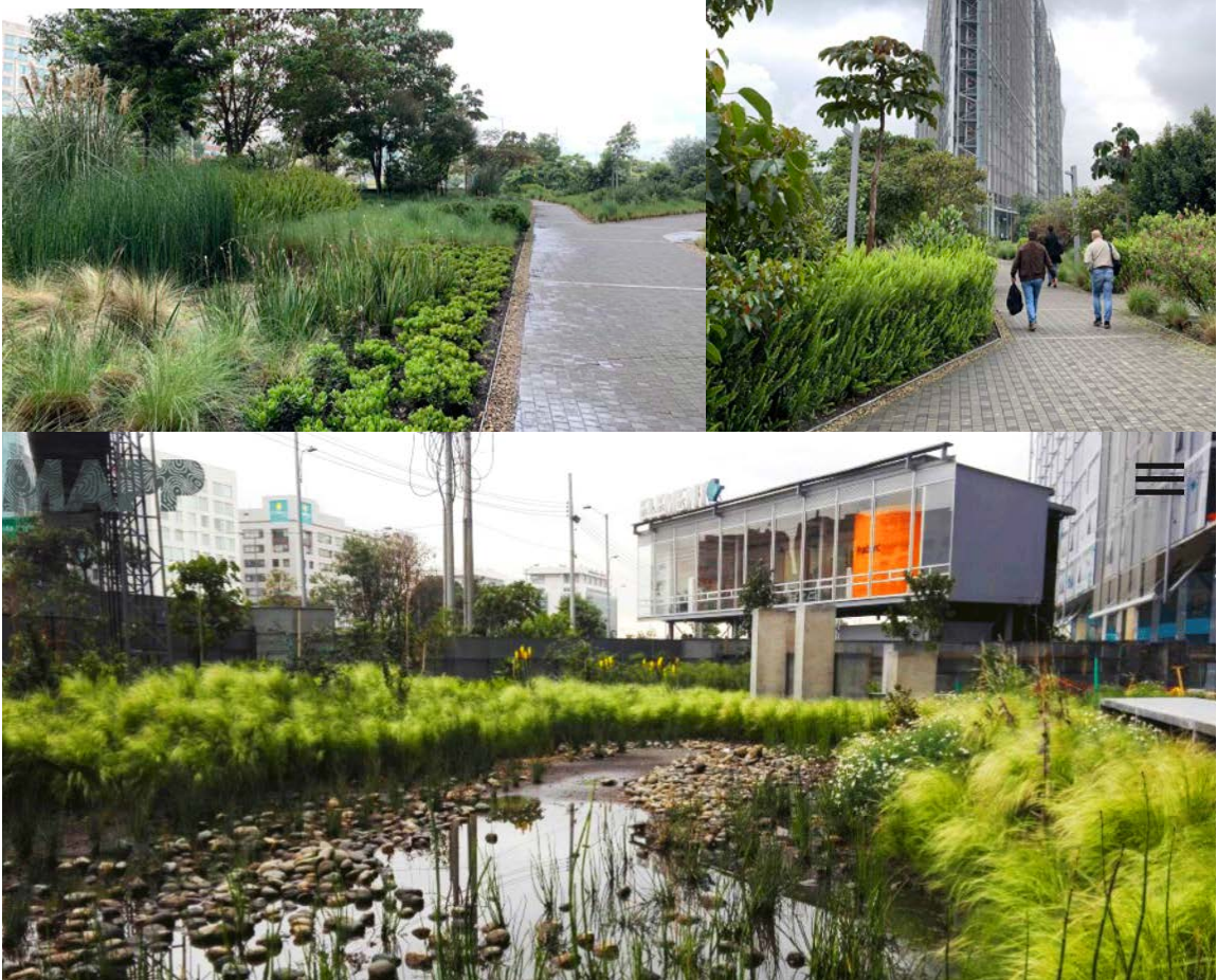
Figure 5.2: SUDS in Elemento Building (69th Avenue and 26th Street), Bogotá, Colombia.
