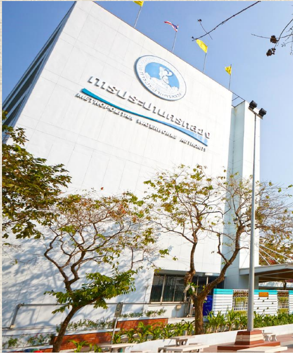
Metropolitan Waterworks Authority (MWA)
