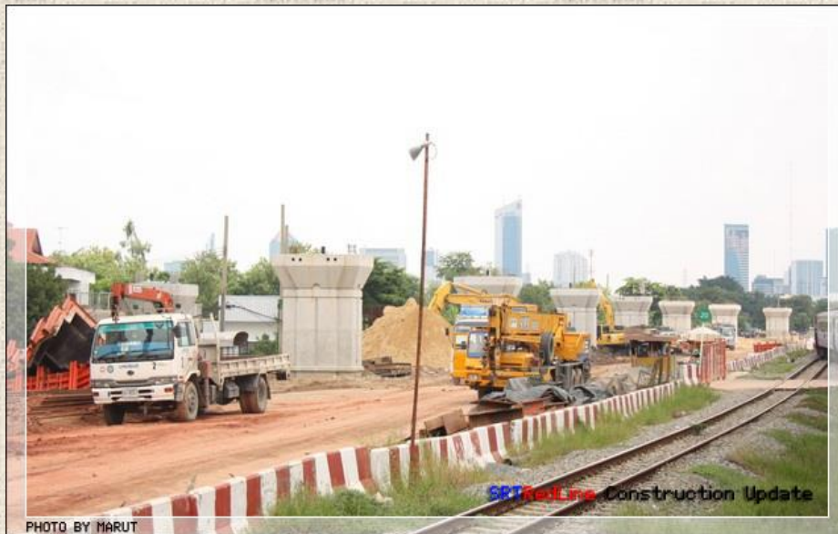
Construction progress of Red line sky train
