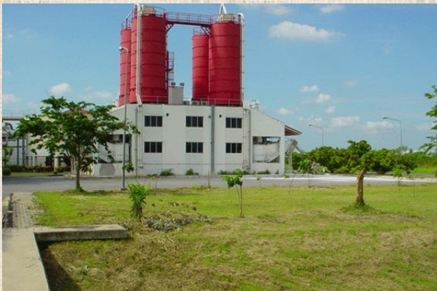
1. Mahasawad water treatment plant
