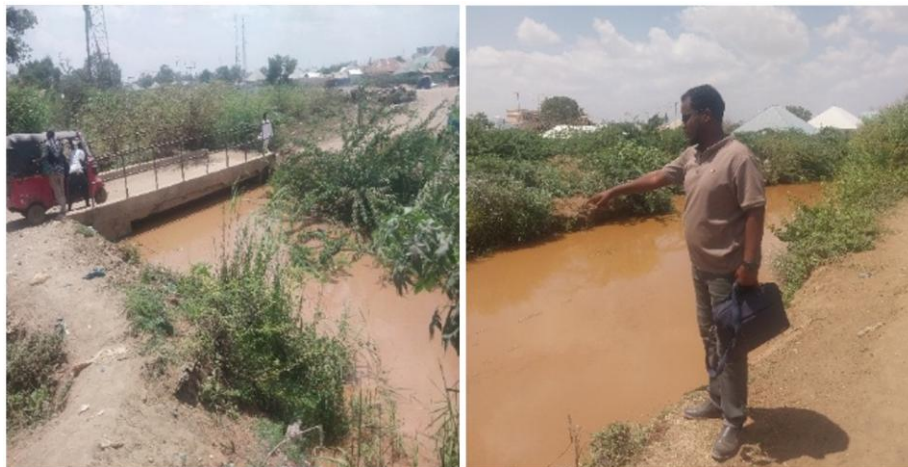
FIGURE 2.4: JOWHAR, IRRIGATION CANALS
