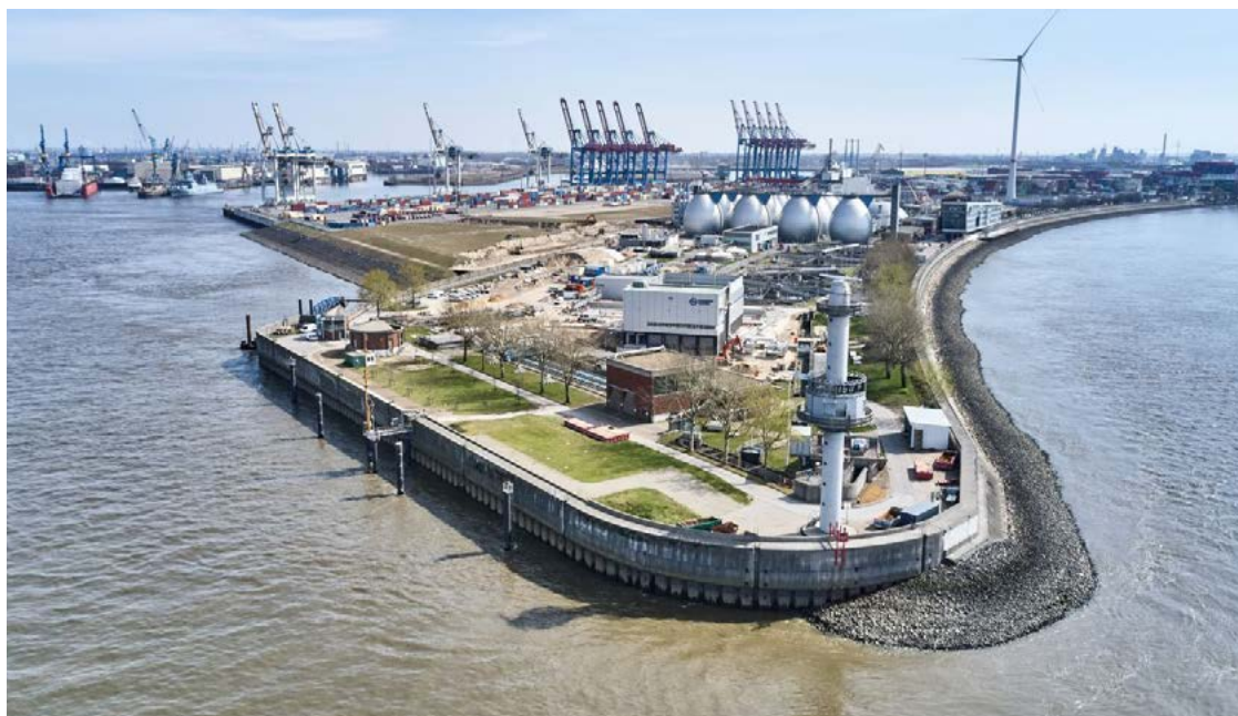
Large-scale centralized wastewater treatment as an energy source in Hamburg, Germany. © Kristina Steiner for Hamburg Wasser
