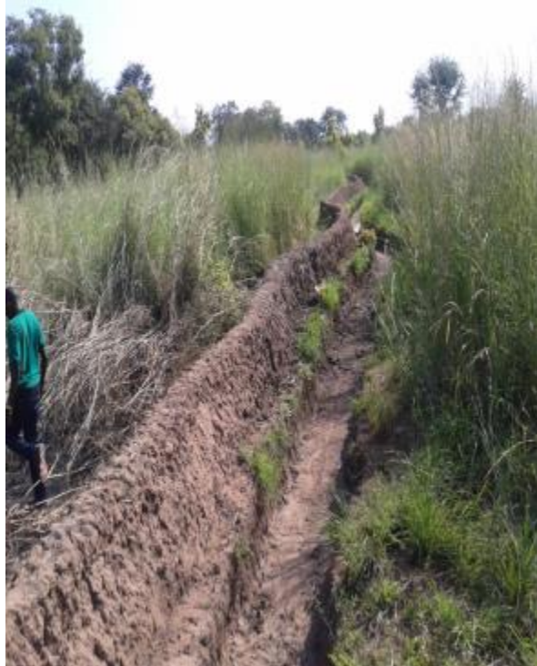
Dykes and drainage constructed by Concern Worldwide Cash for Work beneficiaries in Aroyo
