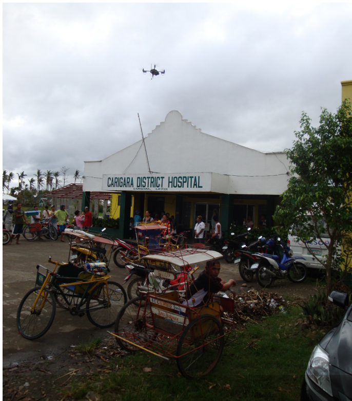
Figure 2 Here the quadcopter drone flies over to survey damage to the local Carigara District Hospital in Tacloban, The Philippines in November 2013.
