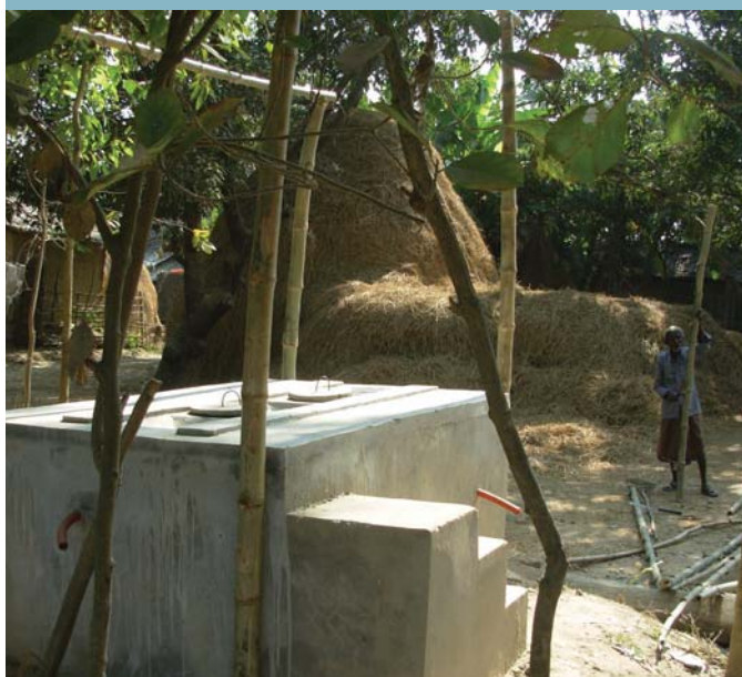
This project in Bihar, India, tackled the financing issue by providing the concrete substructure for flood-resistant toilets, while households were responsible for building the superstructure. Photo: Kim Andersson
