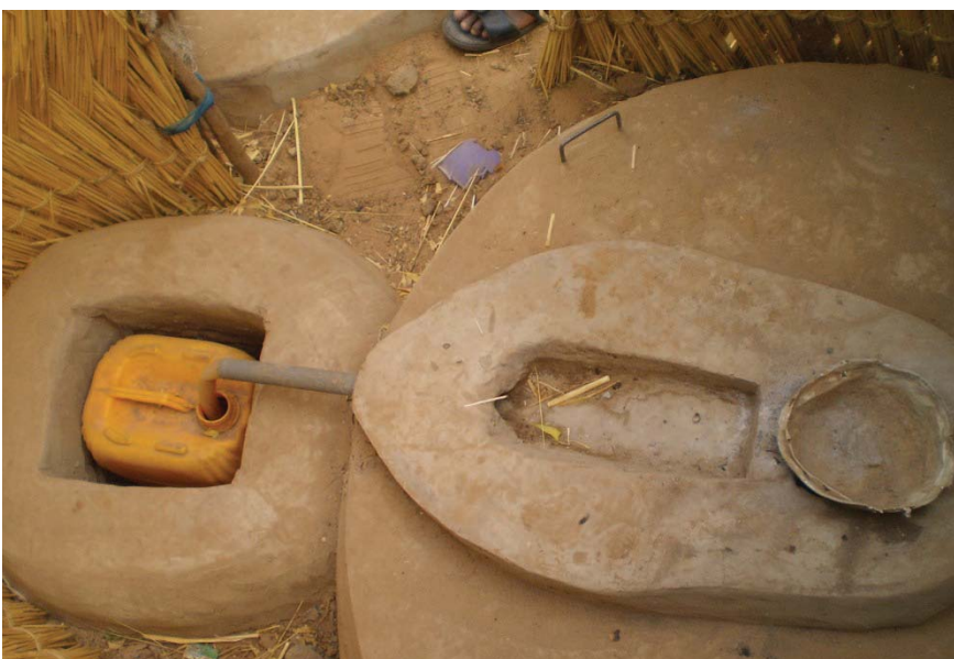
Urine-diverting composting toilet in Niger (left) and a demonstration urine-diverting toilet at the Tarumitra Bio-reserve and Ecology Centre, Bihar, India (right), with rope to facilitate use. Photos: Linus Dagerskog, Kim Andersson.
