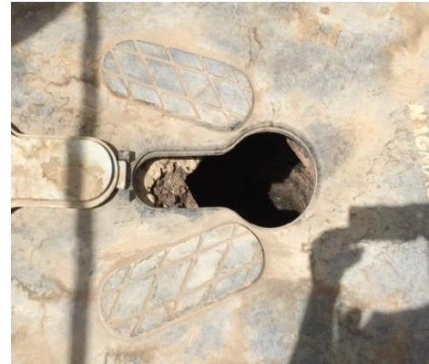
Most of the pit are lined with 3 steel drums of 200L (pit = 600L) which is quite small and impact the lifespan of the pit and the cost of the response.
