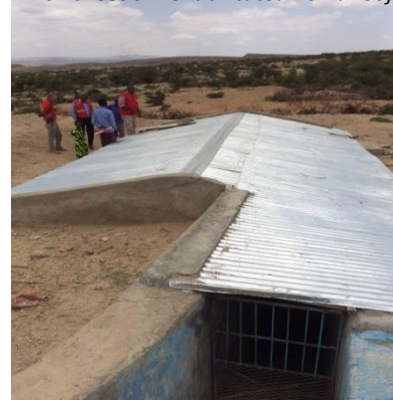
Iron sheet on rehabilitated Berka roof
