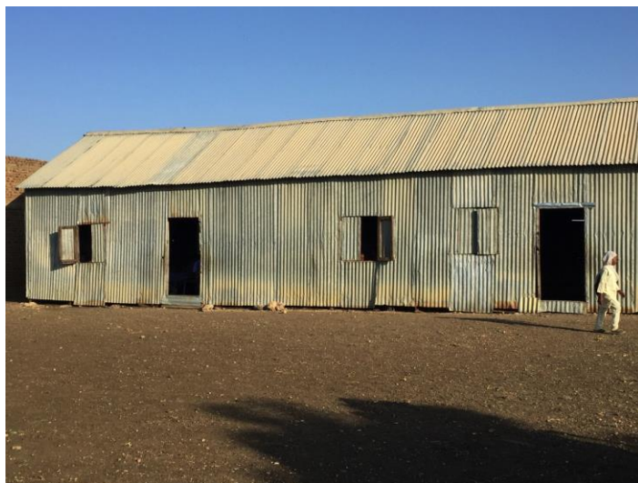
Figure 8 Corrugated School Block, Al Mafaza
