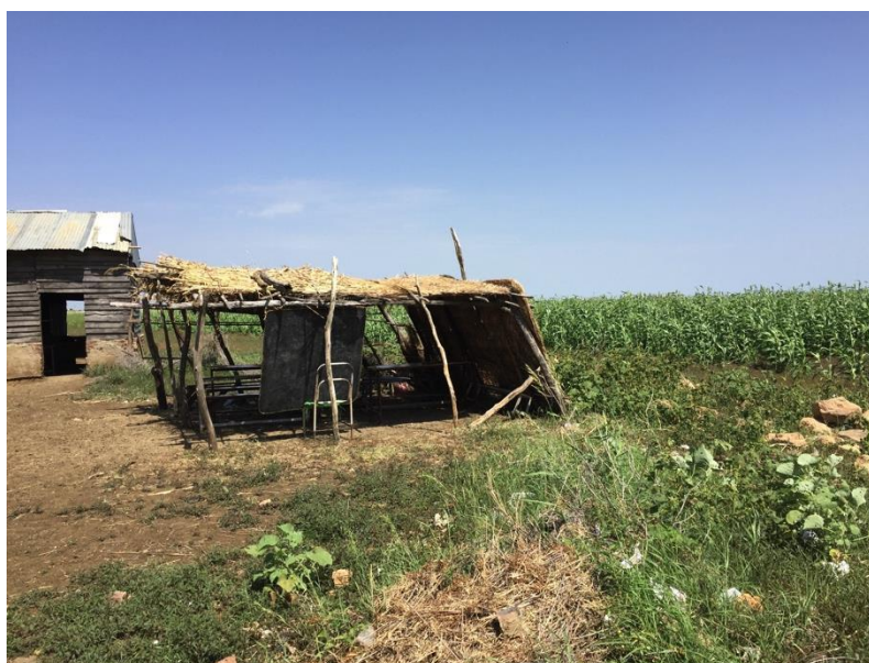
Figure 6 Rakuba Classroom, Al Asama Mixed School, Al Hawata
