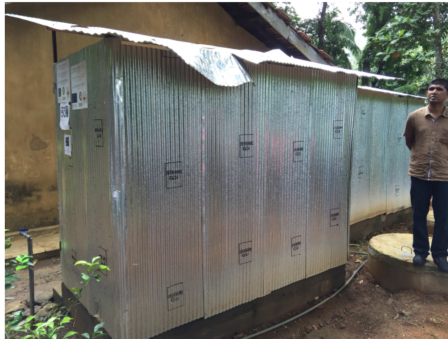
2 latrine blocks with soak pits and a hand washing point
