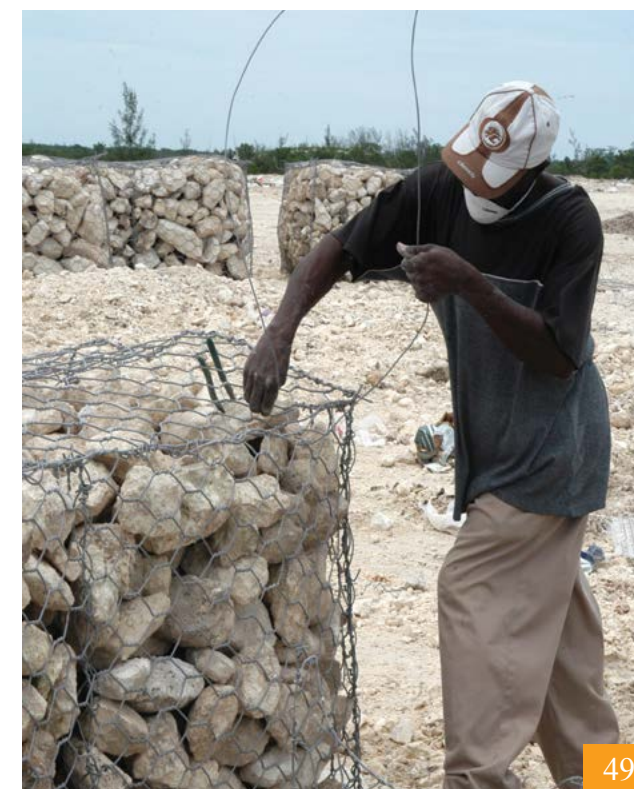
NASSAU, BAHAMS. CONSTRUCTION OF GABION BASKETS. JUNE, 2004
