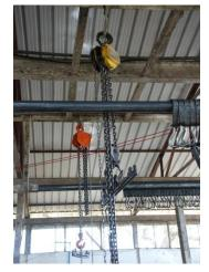
The carcase hanging rail 70 mm diameter steel acceptable condition. The meat hooks are of high quality stainless steel of but require deep remove to cleaning biological debris which could contaminate the carcases.
