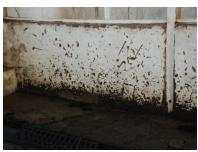
• Much of the she steelwork structure is badly corroded, the floor slab cracked and lifted, drainage channels and grids damaged, the walls were cracked and the walls to floor joints were not sealed.
