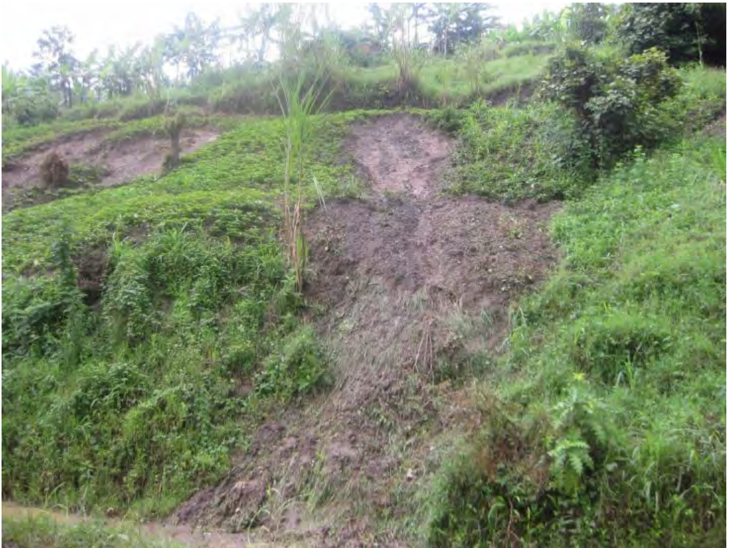
Road embankment soil erosion , Karongi district, Mubuga sector.
