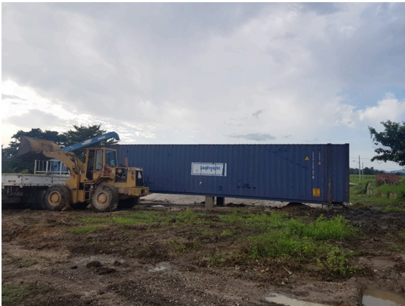
Figure 3: 45' shipping container being hoisted into place Aug 16th, 2017
