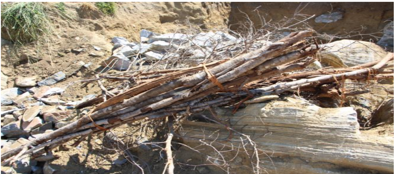
Firewood used as catalyst during rock blasting
