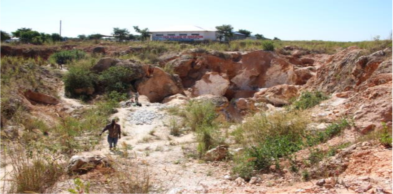
Destabilized terrain and open excavations
