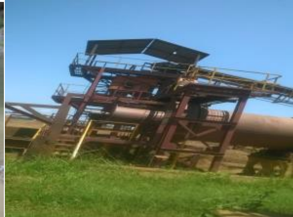
conserved green environment at Namekara mine due to water usage in operations
